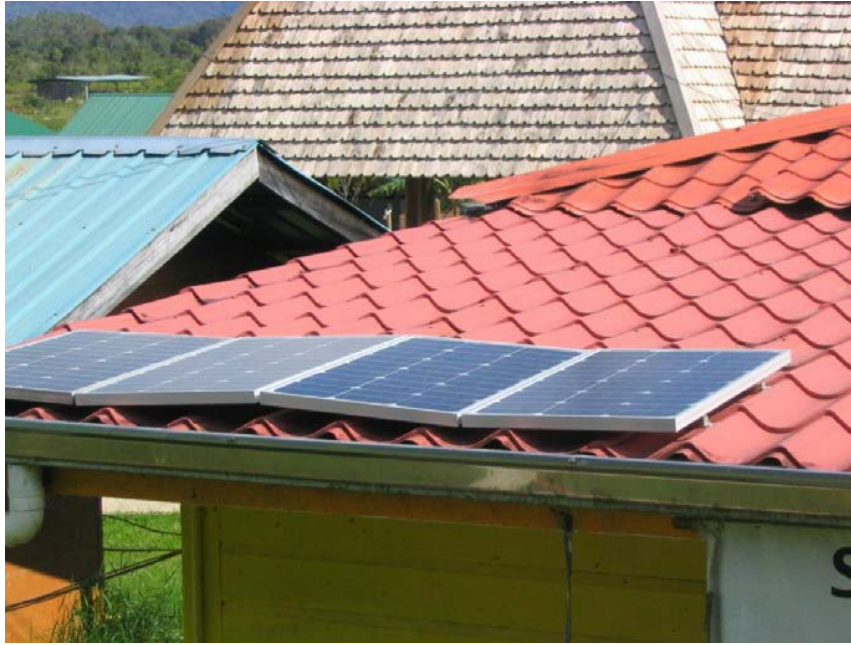
Figure 2-2-4: Solar panel installation on barrio telecentre's rooftop
