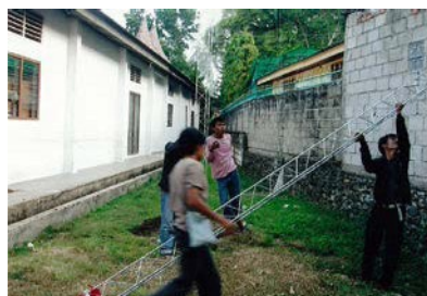
Preparation of Tower Installation
