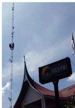
Antenna Unit Installation
